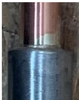
Copper to steel brazed joint
